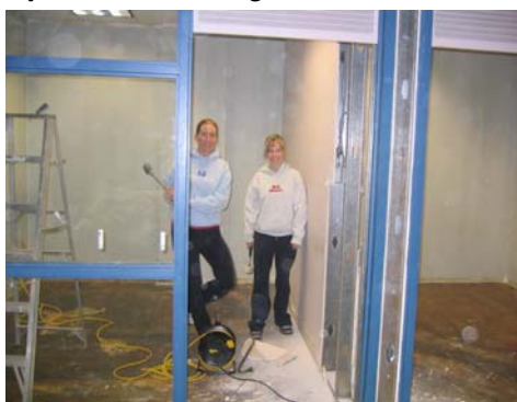
Brenda and Carrie, ready to make the first hole in the wall
